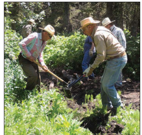
Ron Rassley and Rich Inman work on water barriers
