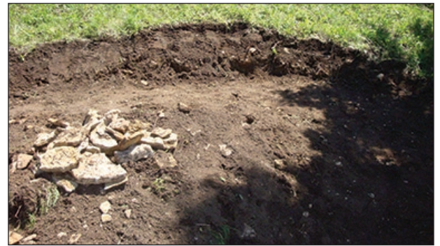
the new switchback, all finished
