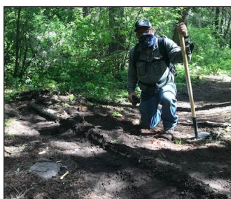
Jim Wing finishing a water bar
