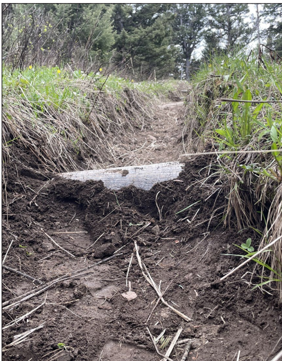
Curt Settergren packing in water bar/steps for trail maintenance
