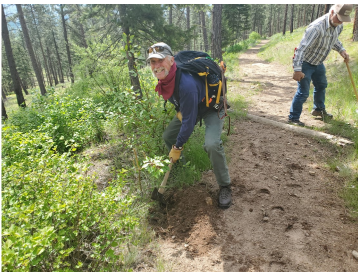
At Larry Creek, Chris Carrera uses a rock hammer to pound in a rebar, Dan Maiyo uses his Pulaski to clear a drainage ditch above a water bar.
