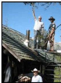
Up on the roof.
