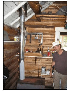
Scott admires the finished chimney job.
