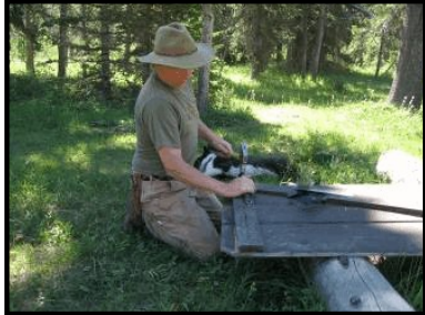
Dan repairs the hay shed door.
