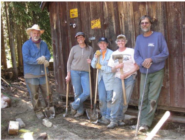
Repairing the barn foundation @ Swet Lake Cabin
