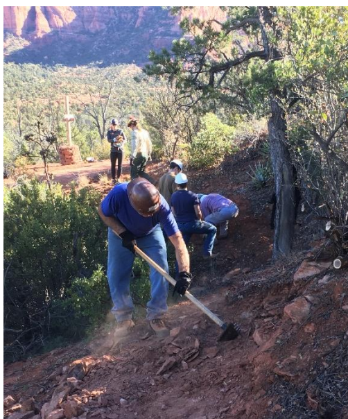
Coconino National Forest: Members of Friends of the Forest alongside other local volunteers help reroute a section of trail to improve drainage, reduce erosion, and decrease future maintenance costs.
