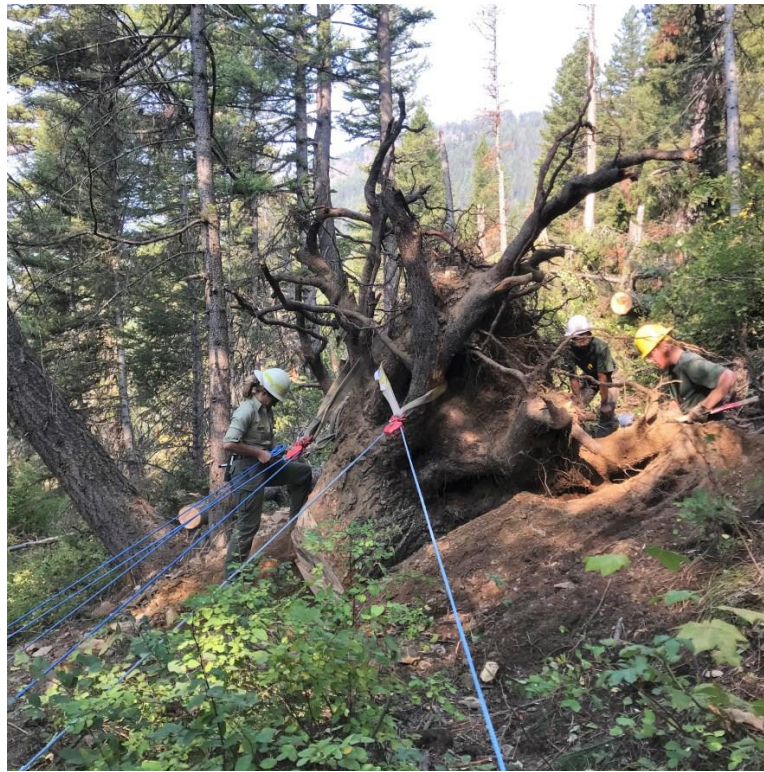
Flathead National Forest: Forest Service employees and Montana Conservation Corps field crews rigging a root ball for removal along the Big River trail on Hungry Horse-Glacier View Ranger District.
